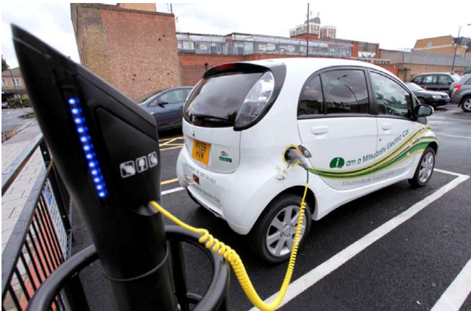
Figure 12: Electric vehicle charging point in Hackney car park
