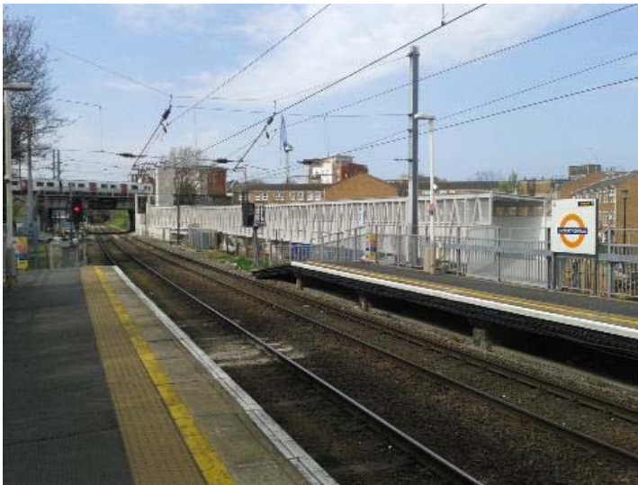
Figure 6: Construction of new Hackney Interchange pedestrian link underway (April 2015)
