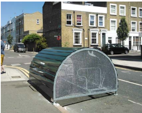
Figure 10: On street cycle hangar in a parking bay
